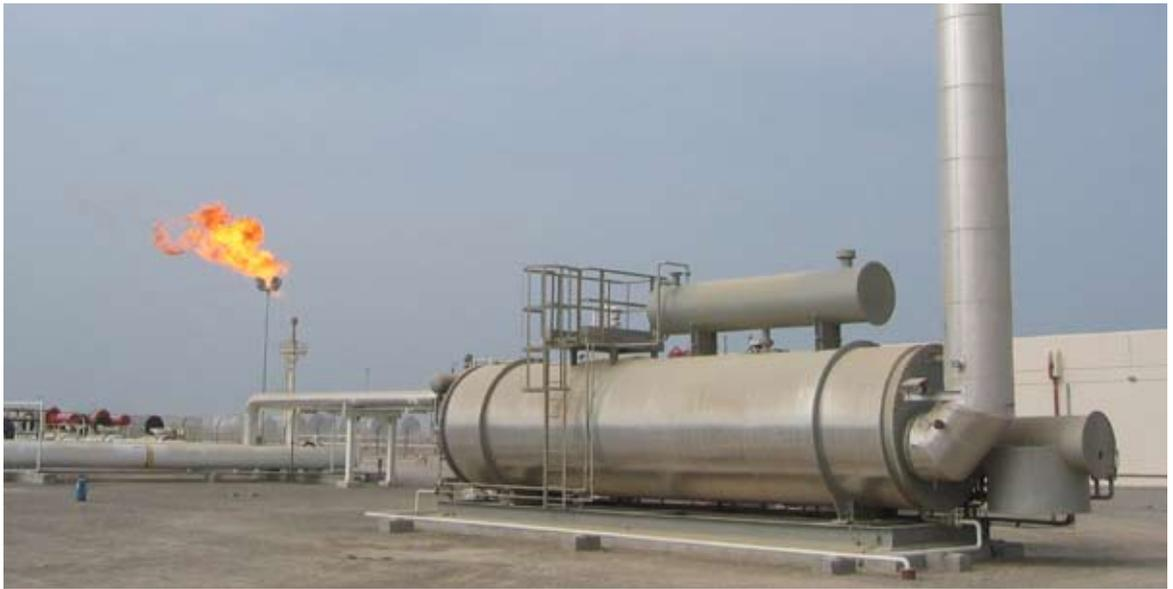
Almost every coil bundle require a tailored design in order to meet the requirements of heat duty, working pressure, corrosion allowance, sour gas service, NACE MR-01-75 and governing specification or normative, usually ASTM or ANSI B 31.3.
